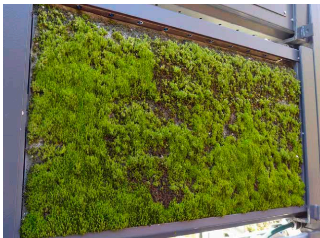
Module of the moss wall on site at the DITF
