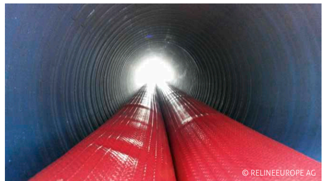
A heat exchange panel within a two-piece sewer pipe
